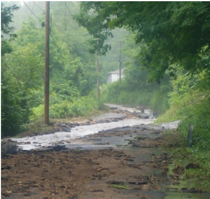
Image 4: July 2021 flooding washed out the road surface along a stretch of O'Neil Road. Photo credit: James McKeon.
