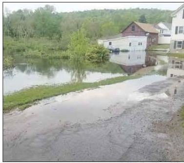
A beaver dam breach caused flooding to this property. Photo Courtesy of James McKeon
